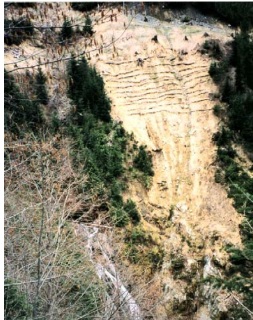
Slope failure associated with logging road construction in the Nanaimo area
